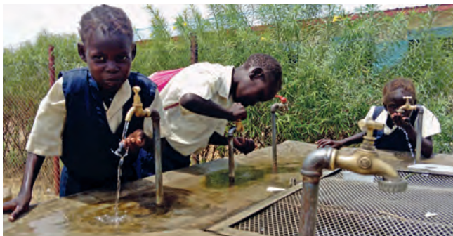
The water pump in Gumbo was repaired with help from Austria.
